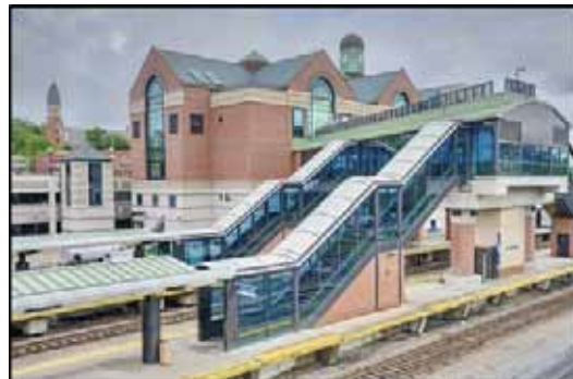
CDTA's Rensselaer Rail Station Station and Boarding Platforms
